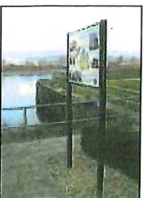
V5. Side mounted posts.
