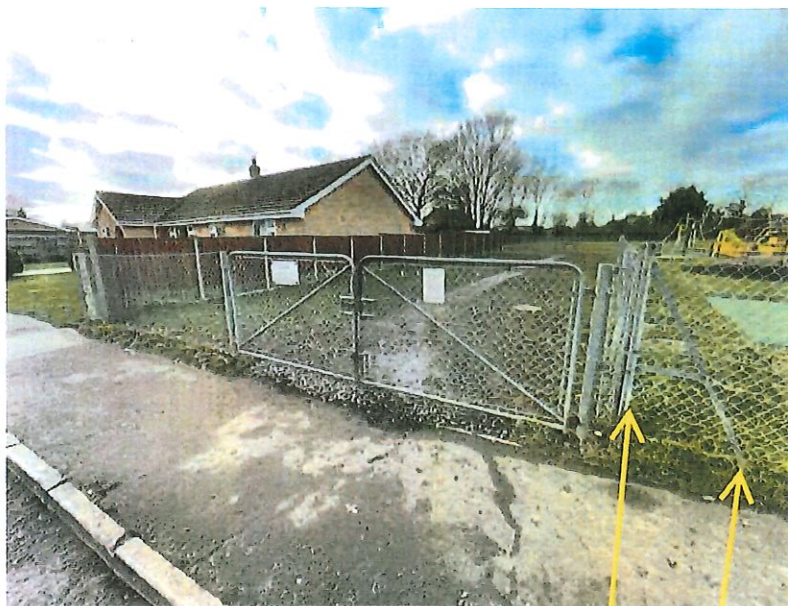
Fence post to stay in place, angled stay to be removed to allow new fence to run off existing post.
